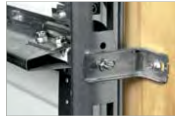
3" commercial grade U-bars provide horizontal stability.
