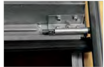
Bottom section roller slide attached to U-bar resists inward and outward force.
